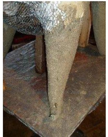
The front leg is wrapped to keep the mortar wet overnight. Additional mortar has been applied to the rear leg on this side.
