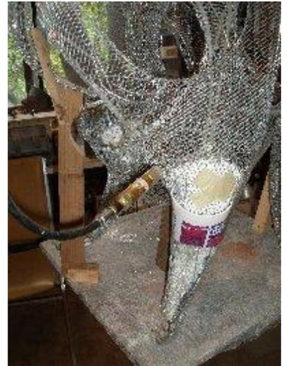
This shows the results of the first application of mortar to the left front leg. It is smoothed to the surface of the expanded metal. Additional layers will get to the finish line.
